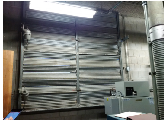
Outside air dampers closed during air handling unit operation
