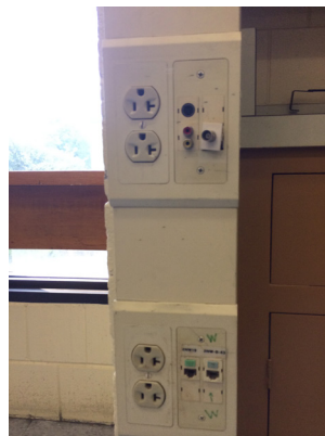
Surface-mounted raceway in classroom
