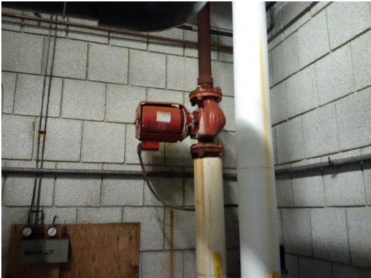
Leaking/corroded in-line pump (pool equipment)
