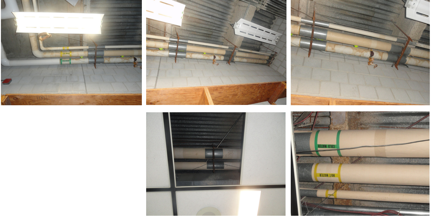
Photo 24: Poor pipe insulation
