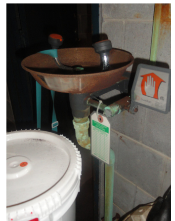
Photo 30: Non-ADA Emergency Eyewash in the Filter Room
