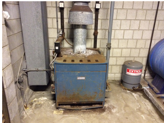
Corroded pool heater
