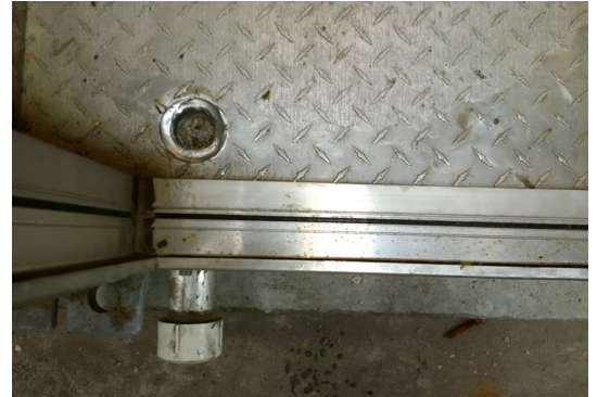
Pool air handling unit floor condensate drain plugged
