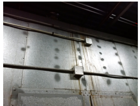
Roof leak on top of air handling unit
