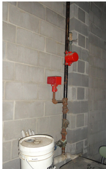
Photo 4: Fire protection components that are not wired
