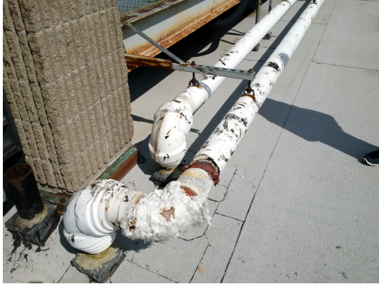
Cogeneration roof-mounted piping damaged insulation and roof flashing
