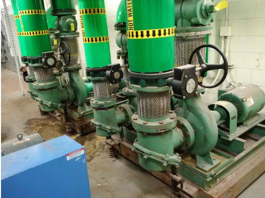
Hot water pumps bulging flexible connections
