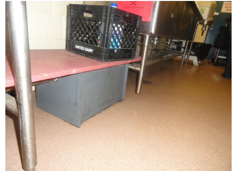
Photo 6: Grease trap at triple pot sink
