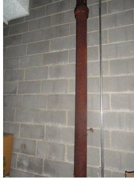
Photos 25: Existing rusted/corroded storm piping
