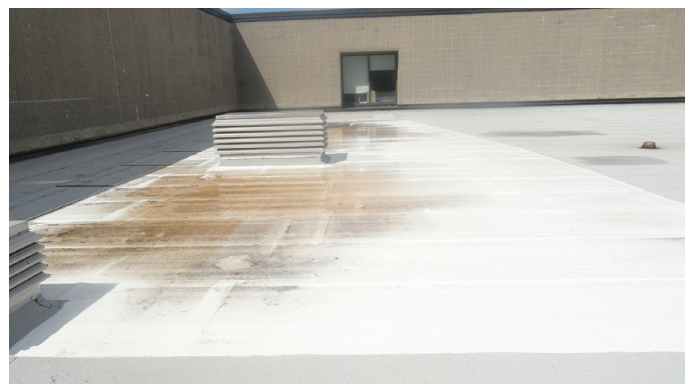
Photo 16: Ponding Issues on the roof
