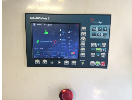
Cogeneration control panel showing active alarm mode
