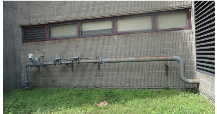
Photo 5: Gas Service, Gas Meter and Piping
