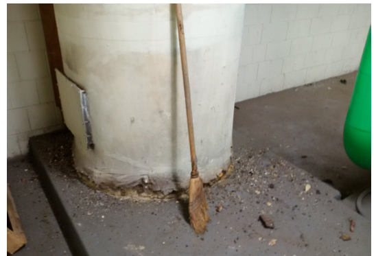
Flue damaged insulation
