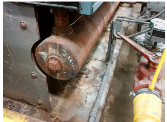
Boiler header showing rust
