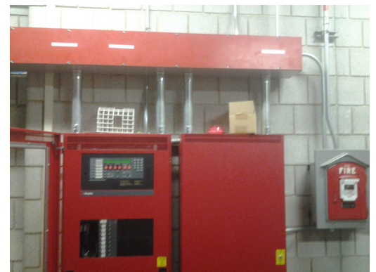
Existing FACP, master box and associated equipment
