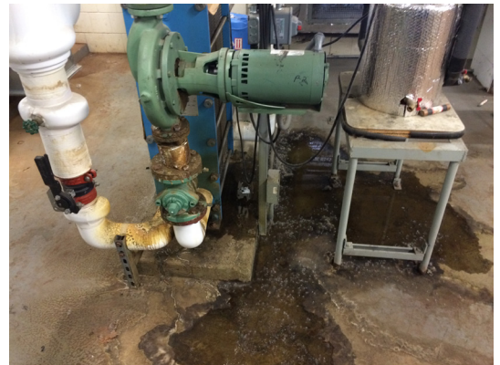
Cogeneration in-line pump, piping, valve leaks
