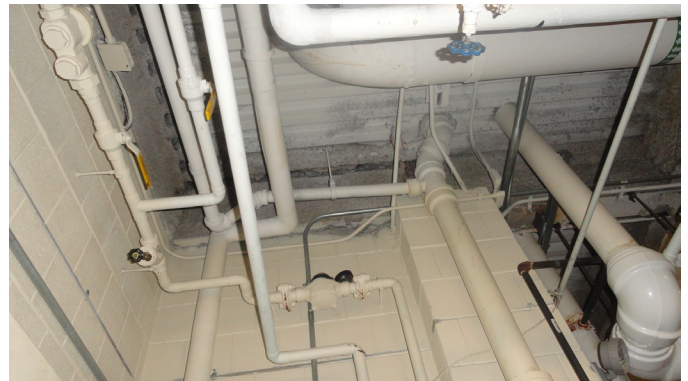
Photo 1: RPBP and Water Meter for HVAC Make-Up
