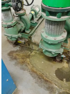
Hot water pump leaks
