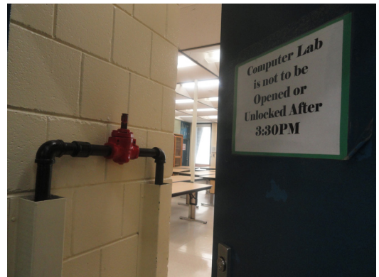
Photo 10: Exposed gas valve
