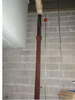
Photos 25: Existing rusted/corroded storm piping
