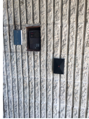
Video intercom and card reader at front entrance
