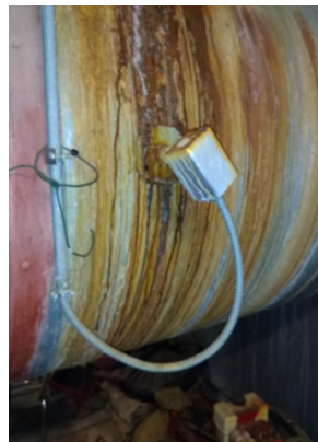
Non-insulated ductwork leaks
