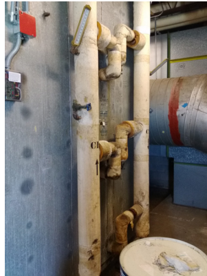
Piping damaged insulation
