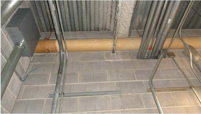
Photo 13: Wet pipe installed above Electrical Panels
