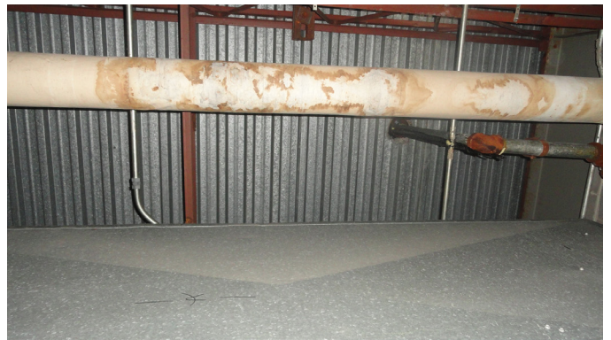
Photo 12: Pipe Insulation in poor condition
