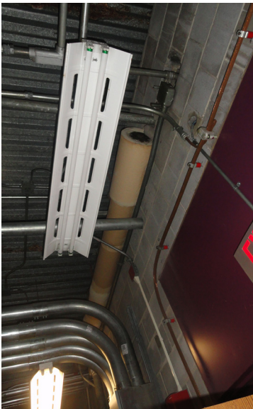
Photo 13: Wet pipe installed above Electrical Panels
