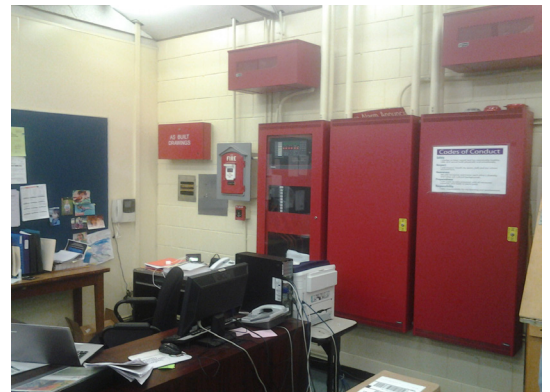
Existing FACP and associated equipment
