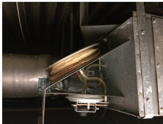
Terminal unit damaged actuator
