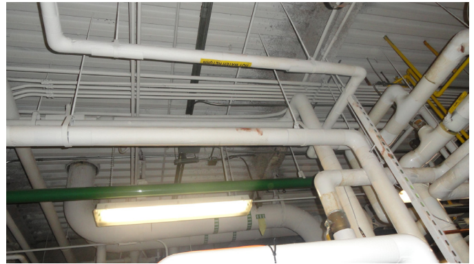
Photo 3: Damaged PVC jackets and pipe insulation
