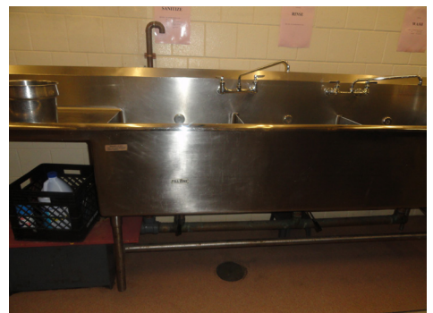
Photo 7: Waste Piping Installation at Triple Pot Sink
