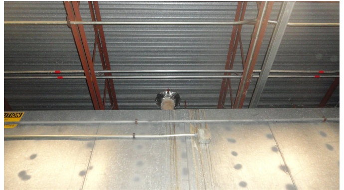
Photo 11: Leaking Roof Drain
