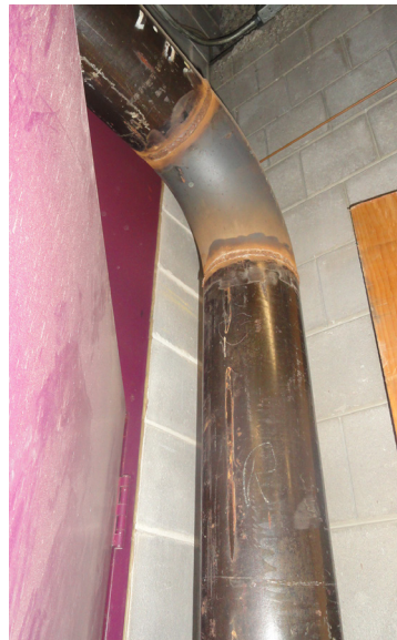
Photo 13: Wet pipe installed above Electrical Panels
