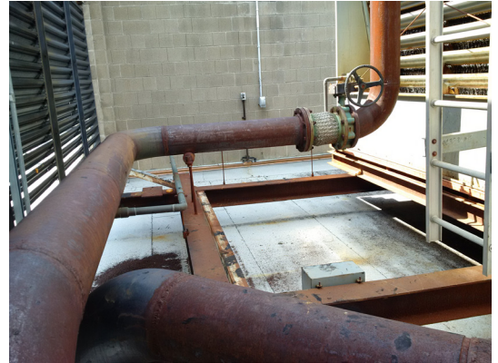
Insufficient condenser water piping support at cooling tower
