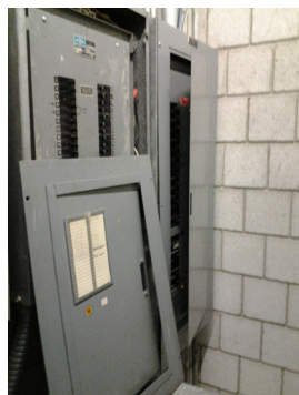
Examples of original panelboards in poor/failing condition
