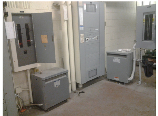
Example of "emergency power" equipment installation (no ATS found)
