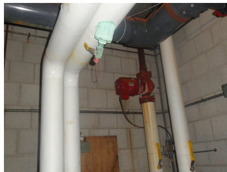
Photo 29: Leaking pump in the Filter Room
