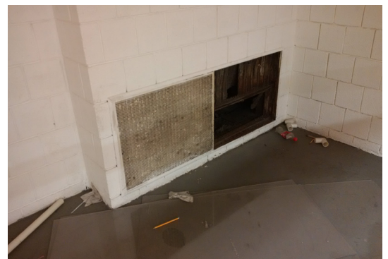
Small gym air dirty/missing register
