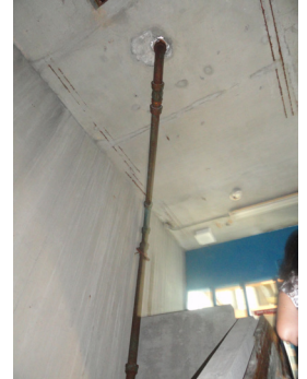
Photos 26: Existing rusted/corroded piping
